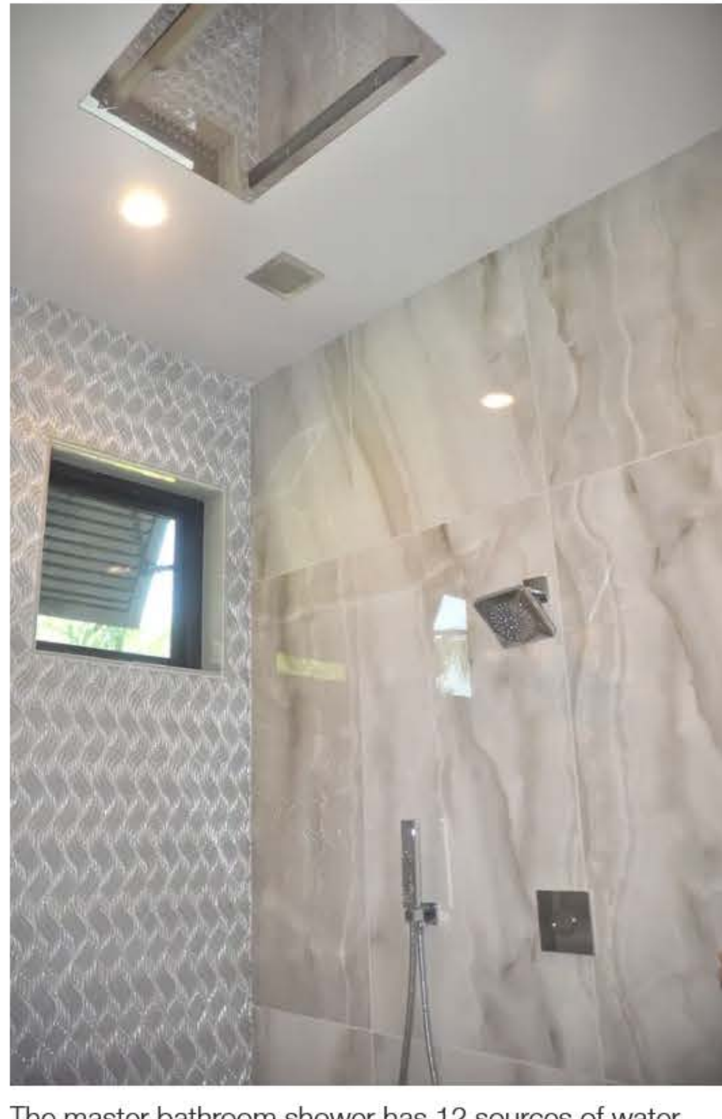
The master bathroom shower has 12 sources of water including a rainhead and many side sprayers. There are no faucet handles. Instead everything from water flow to temperature is controlled by little computer screens. The computers also control the music from the speakers in the shower. Photo By Andrea Stetson
