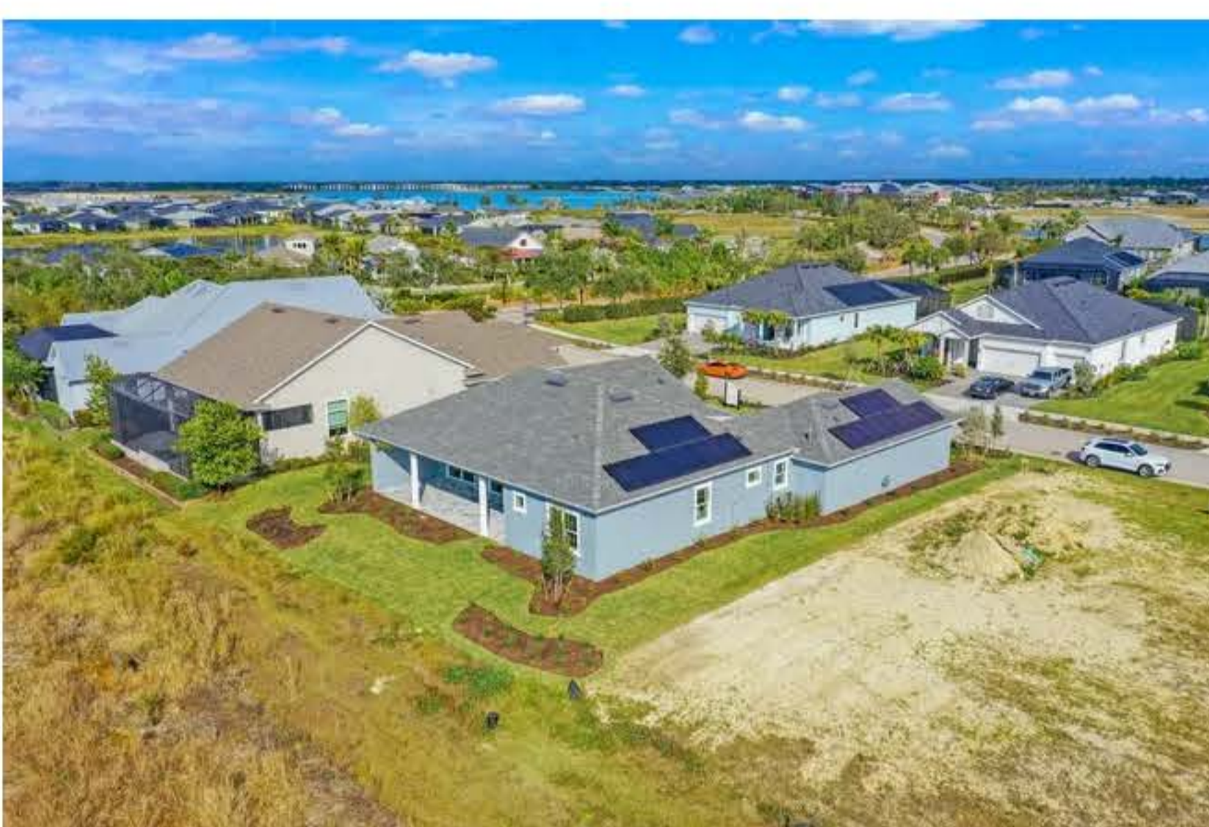
The Annette has solar panels on the roof, duct work that is under air, landscaping, design and more to make it a Net Zero home. Florida Lifestyle Homes hopes to build more net 0 houses in the future. Photo From Florida Lifestyle Homes
